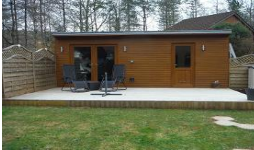
View of building as seen from the applicants garden.
